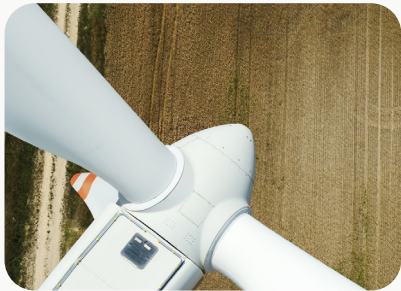
Renewable energy Solar and wind farms & battery energy storage systems.
